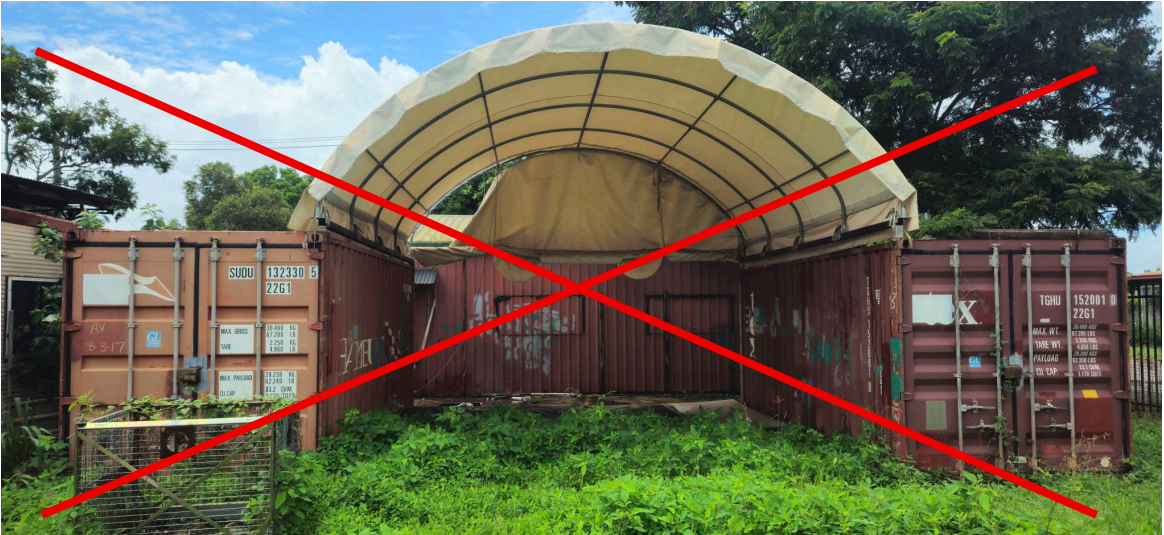
14 * Arched fabric cover + two 6m shipping containers
