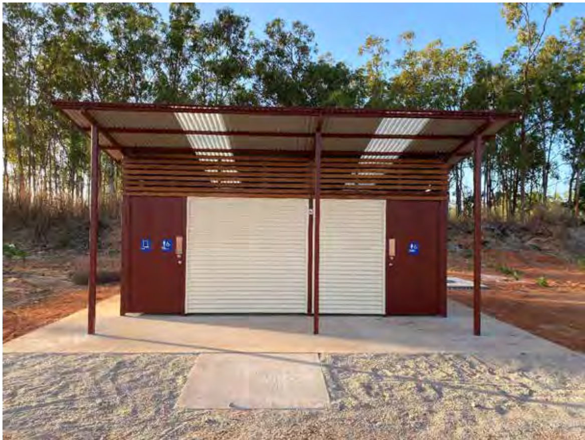
New facilities constructed at Aak Ngench Thayan Cemetery.
