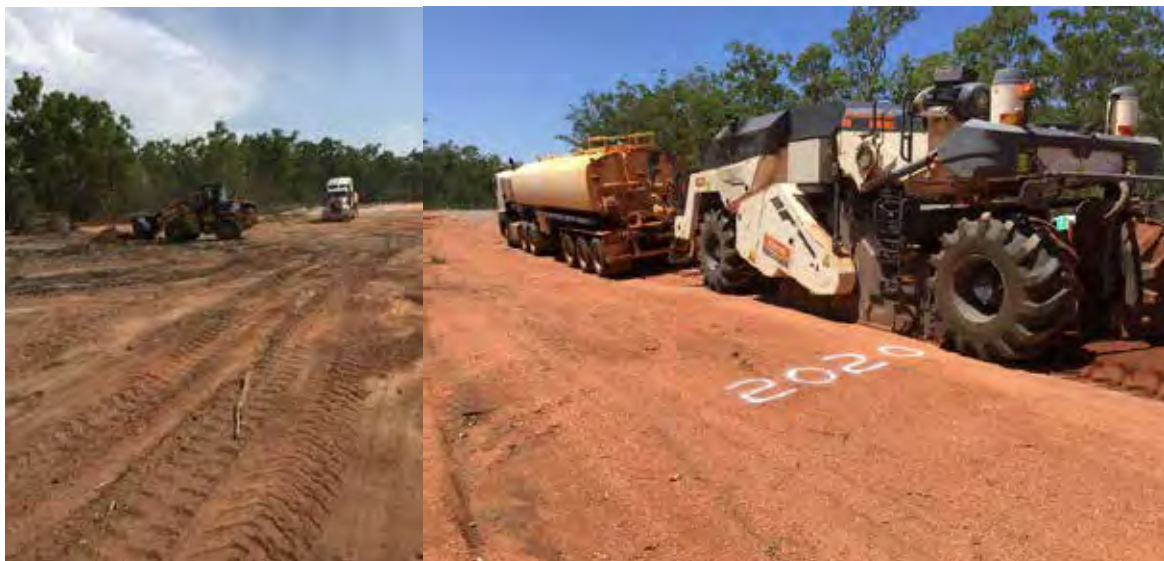
Ngaay Road Industrial Estate Aurukun Access Road
