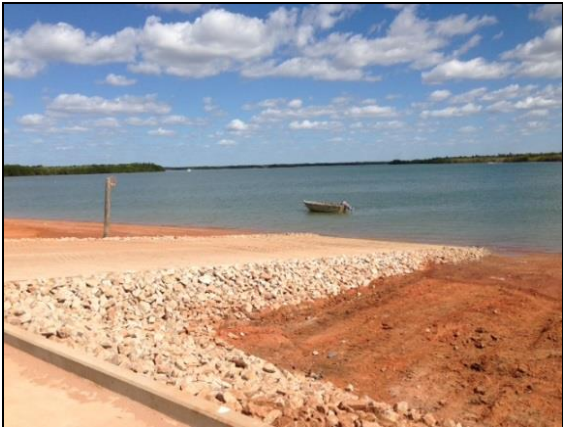
Barge Landing Project (now completed)
