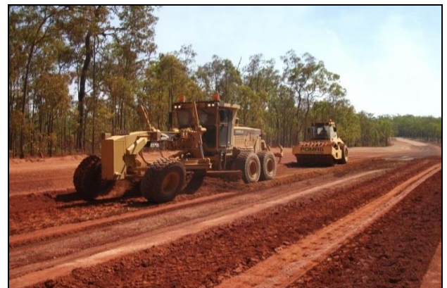
Ongoing Road Maintenance
