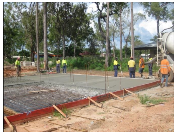
Project Construction continues
