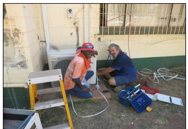
Electricians on the job
