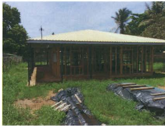
House under construction
