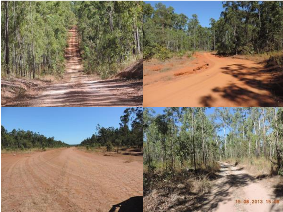
Figure 2-1 Typical condition of the existing running surface
