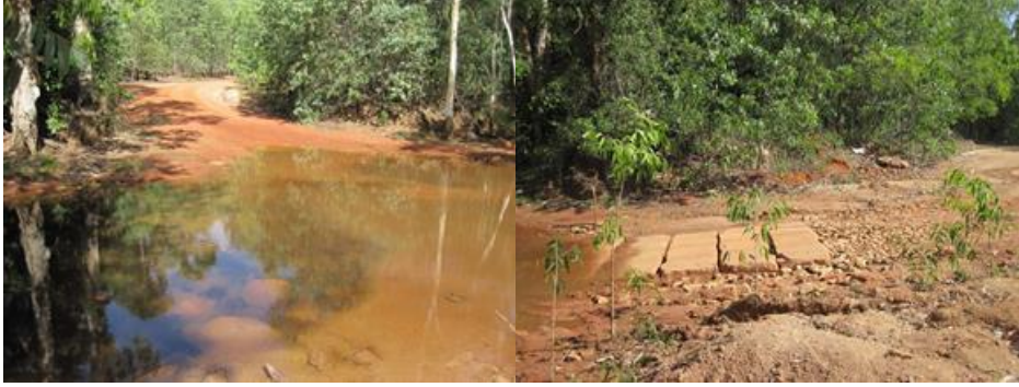
Figure 3-17 Coconut Creek crossing during flow
