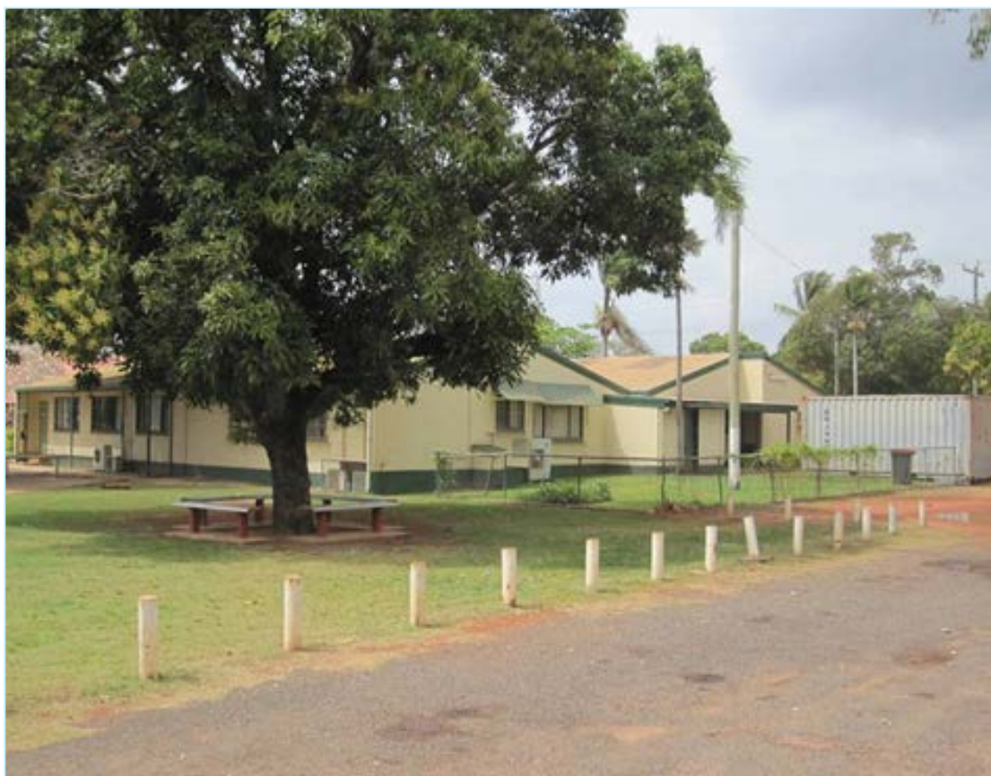
Image 11 – Aurukun’s Council administration building
