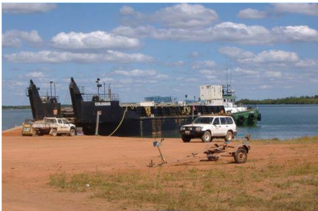
Image 10 – The Aurukun barge ramp
