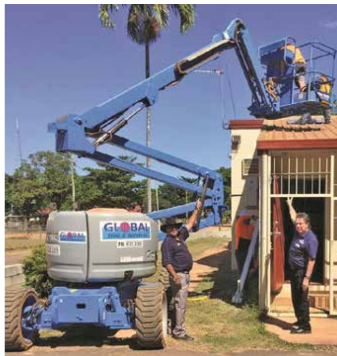
Mayor Dereck Walpo & CEO Bernie McCarthy, CCTV Installation - Shire Office Building
