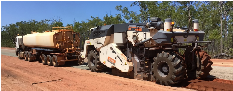
Aurukun Access Road Upgrade
