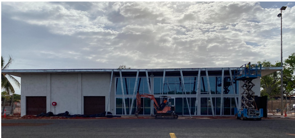
The upgraded Airport Terminal, expected to be officially opened in October 2021
