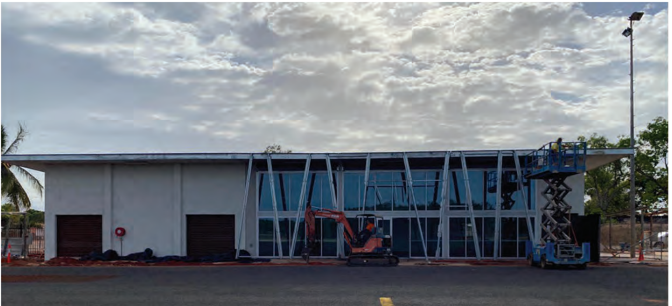
The upgraded Airport Terminal, expected to be officially opened in October 2021
