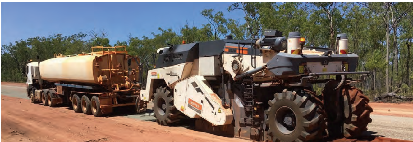
Aurukun Access Road Upgrade
